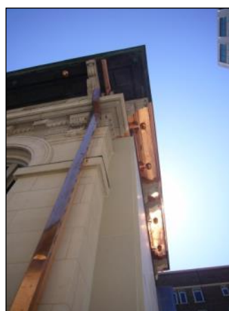
Every effort should be made to preserve historic buildings. This picture shows the preservation of a historic structure where damaged or missing historic materials have been replaced with matching materials.
