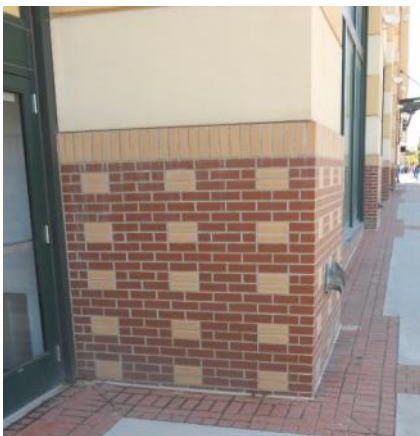
Brick, stone and other durable materials are required on the first floor of buildings.
