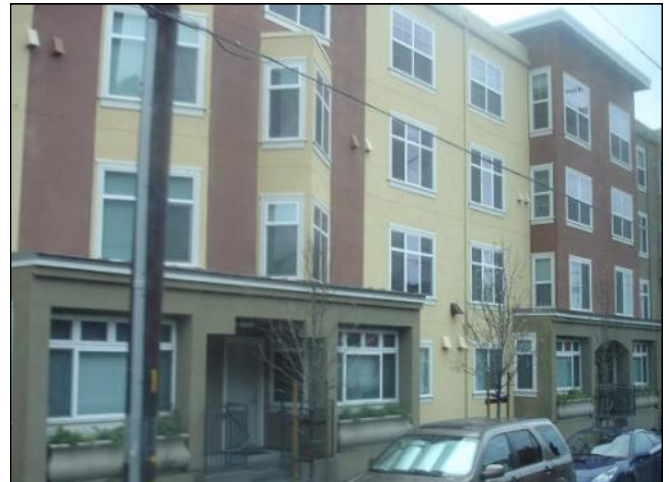
This affordable residential building provides dwelling units of various sizes to accommodate different household sizes.
