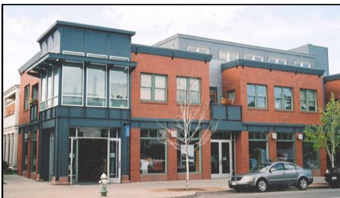
This building includes an entrance on the corner.
