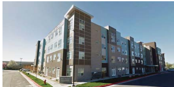
West Station Apartments 175 N Harold Street
